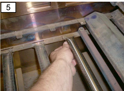
For Standard Input Models, pull the hitchpin from the burner mounting flange.
